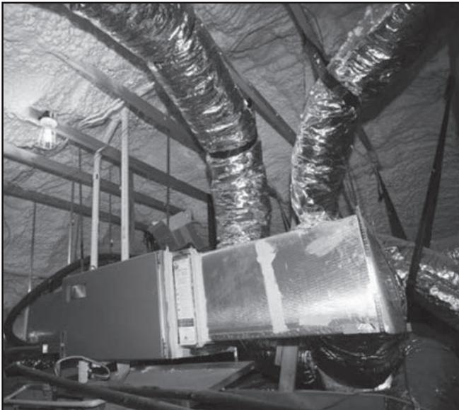
Figure 11. Moving ducts within the conditioned space results in savings for hot climates. Figure courtesy Ren Anderson, National Renewable Energy Laboratory (NREL).
