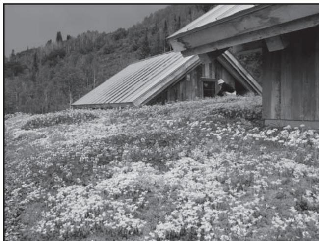
Figure 14. A green roof located in Steamboat Springs, Colorado, taking advantage of native plants in its design. Designed by Lisa Lee Benjamin and Andy Creath, built by Green Roofs of Colorado. Photo courtesy Lisa Lee Benjamin.
